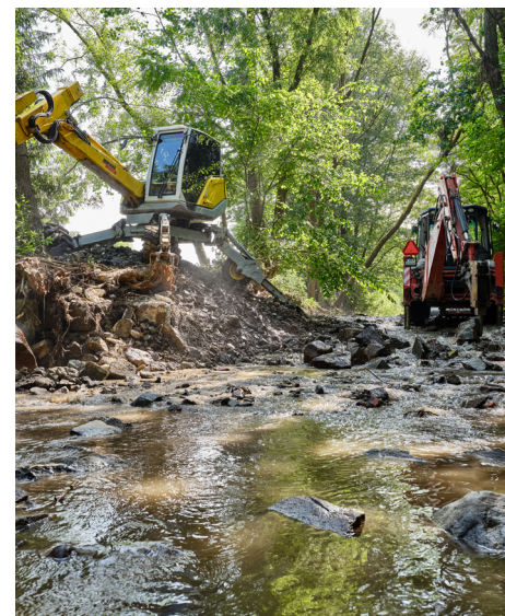
Hučava weir removal, Slovakia, 2021. © Rob Kleinjans
